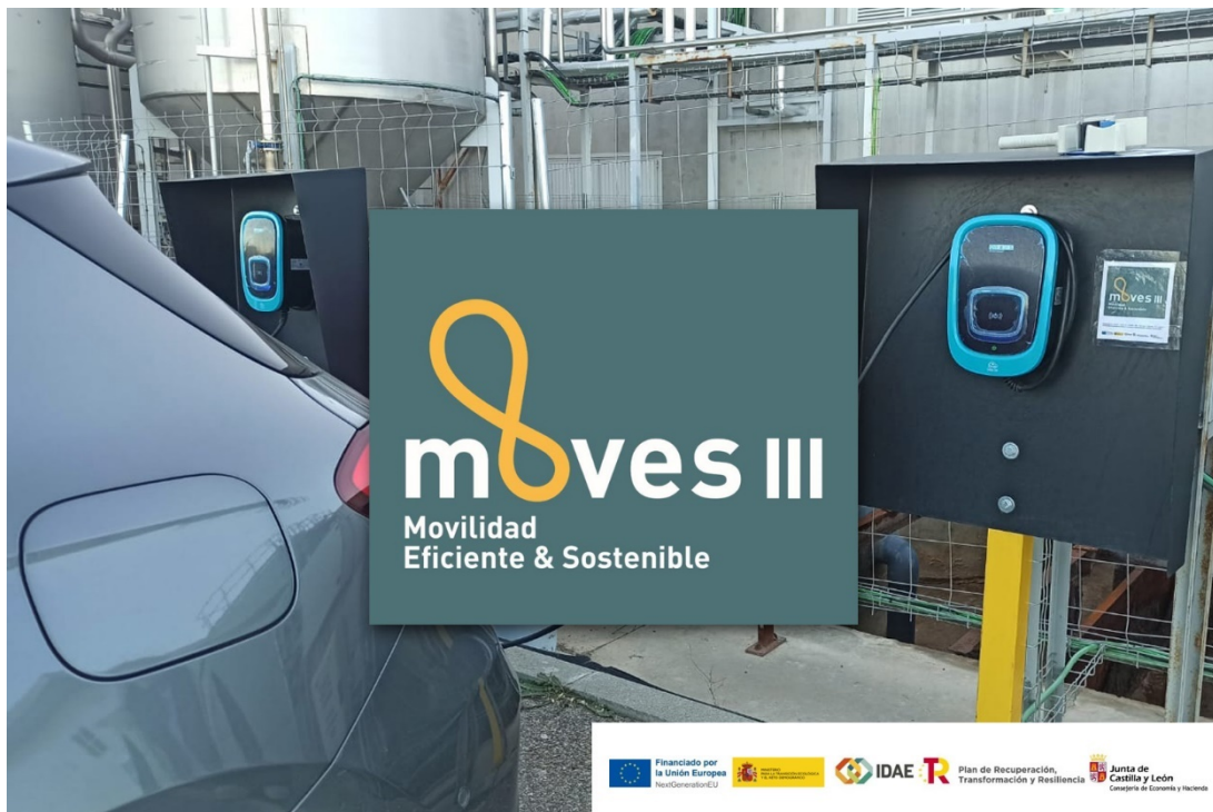
Figure 2 MOVES III EV charging point installation
